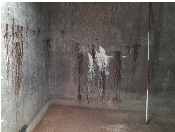
Figure 5: Deterioration within the bunker.
